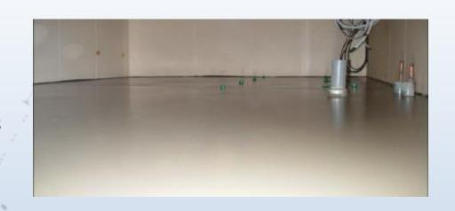
DURASTIC SOLASDEK LIGHTWEIGHT A60 DECKING is an "A" class fire resisting horizontal division of A60 standard for cabins, alleyways, public rooms, control areas etc. Approved floor coverings such as Carpet, Linoleum, Vinyl, Rubber & Epoxy Systems can be the finish. It also provides a suitable base for Ceramic and Mosaic Tiles & Epoxy Systems in wet spaces such as galleys, toilets, wash places etc. Ideal for LQs with weight restrictions.
